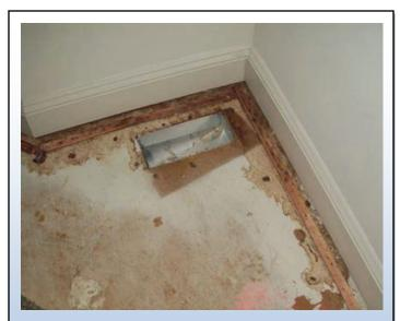
Photo 2: Staining on the subfloor in the area shown in photo 1 clearly indicates that the water infiltration was coming from the wall cavity. There was no discoloration around the supply vent that would indicate that the discoloration on top of the carpet was mold growth from water on all sides of the register.
