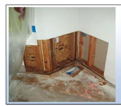
Photo 3: Removal of the mold impacted drywall revealed the new sheathing board that had been installed during the exterior portion of the remediation project. Removing the blown-in and cellulose insulation from the outside and later replacing it with foam board insulation substantially reduced the amount of mess and cleaning that was necessary during the interior phase of the remediation.
